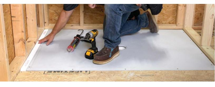
Pre-pitched to match pan surface and support pan water drainage.
