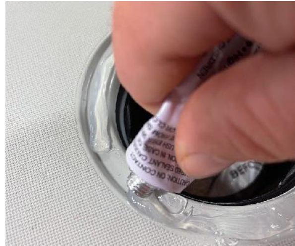
Apply a small bead of silicone to recessed flange
