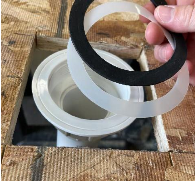
Teflon gasket then rubber gasket
