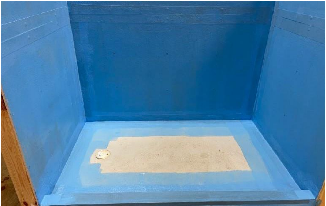
After 1 coat of waterproofing (somewhat transparent)
