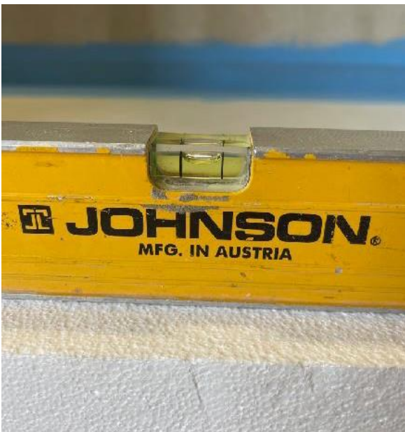
Make sure the curb is level
