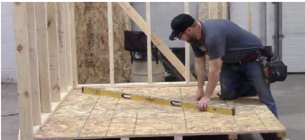
Check subfloor for level & flatness
