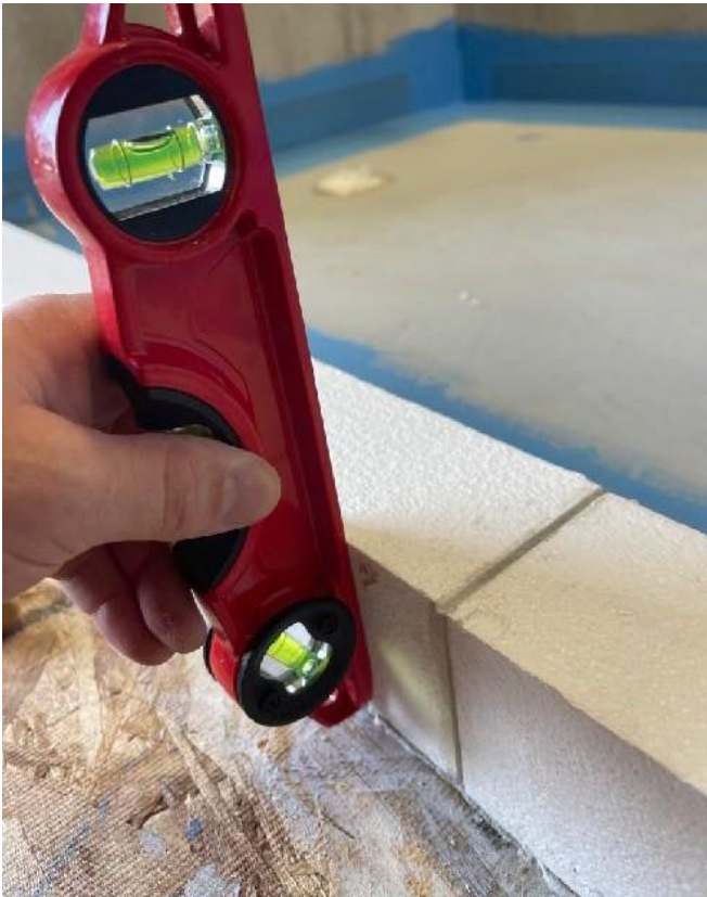
Check face of the curb for plumb
