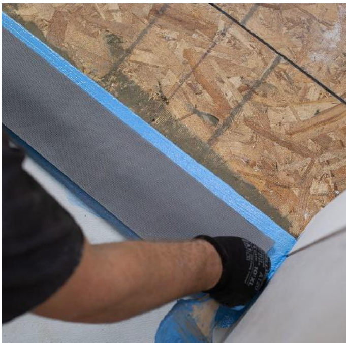
Embed tape on the top of curb first
