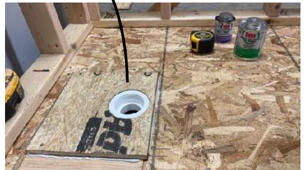
Drain support block installation
