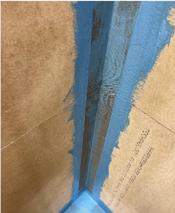
Vertical inside corner embedded
