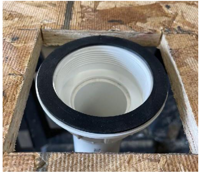
Rubber gasket will always contact the pan
