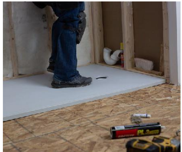
Apply body weight throughout the pan
