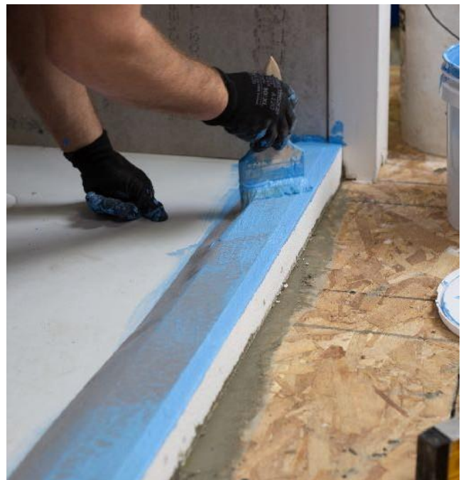
Coat over the tape on top of the curb
