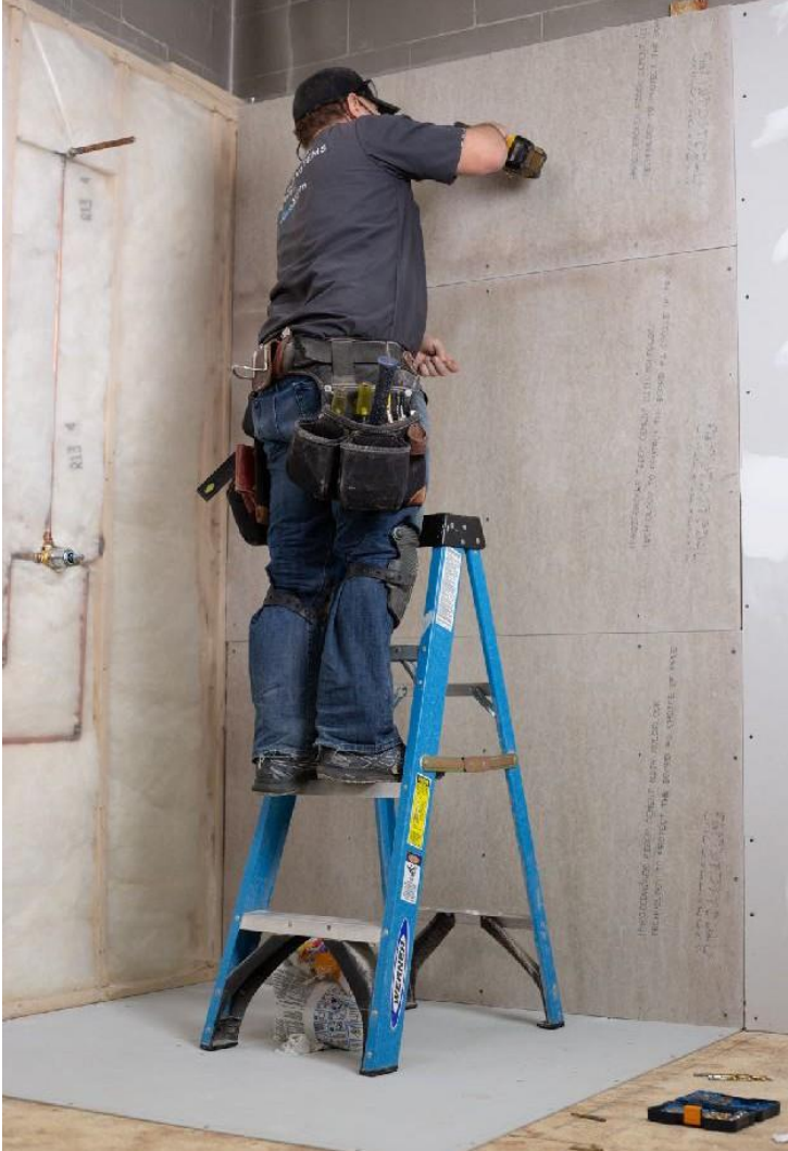
Install tile backer on walls and floors
