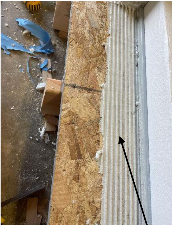
Apply 1/4" notch to substrate
