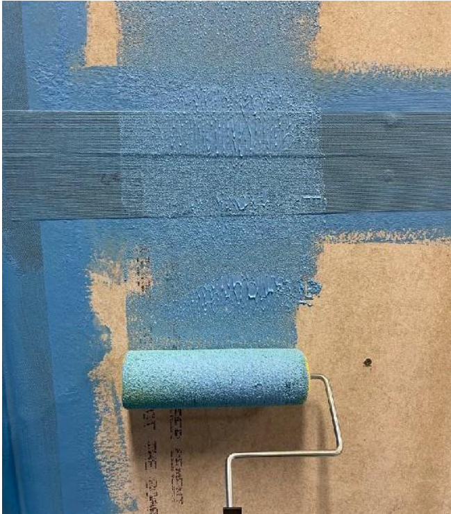
Apply first coat in either a vertical or horizontal direction
