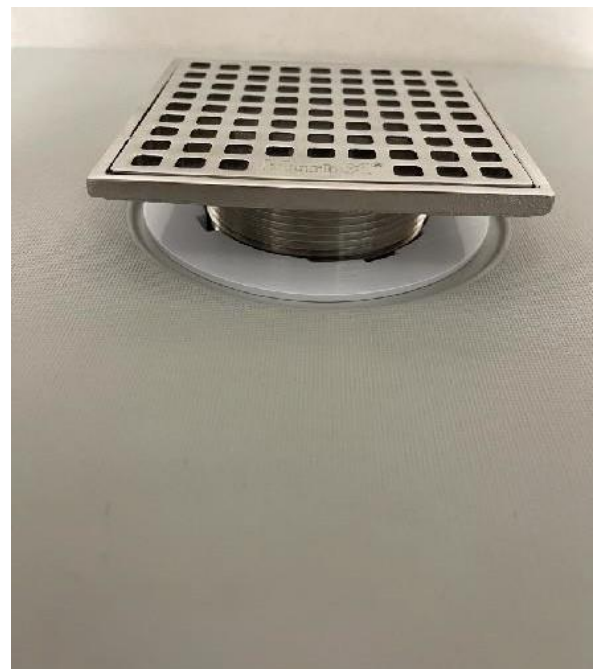
Drain riser threaded into double threaded nipple after connection to pan
