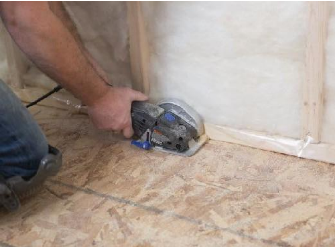
Use Dremel Ultra Saw with flush cut blade against wall plates
