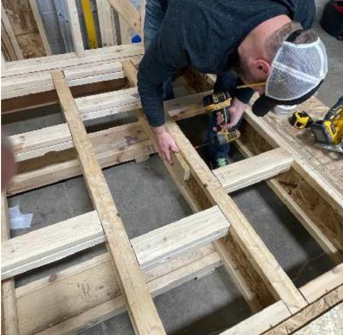
Cleat with notched side up to fit I-joist
