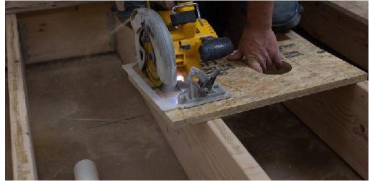
Cut 1-2" strip off leftover drain support block for spacer
