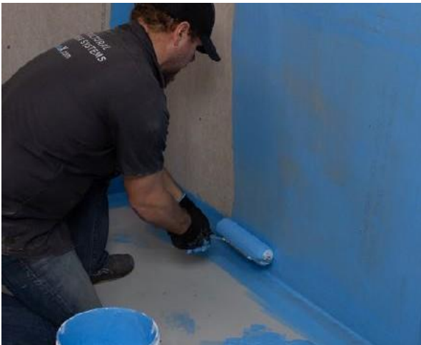
After 1 coat of waterproofing (somewhat transparent)
