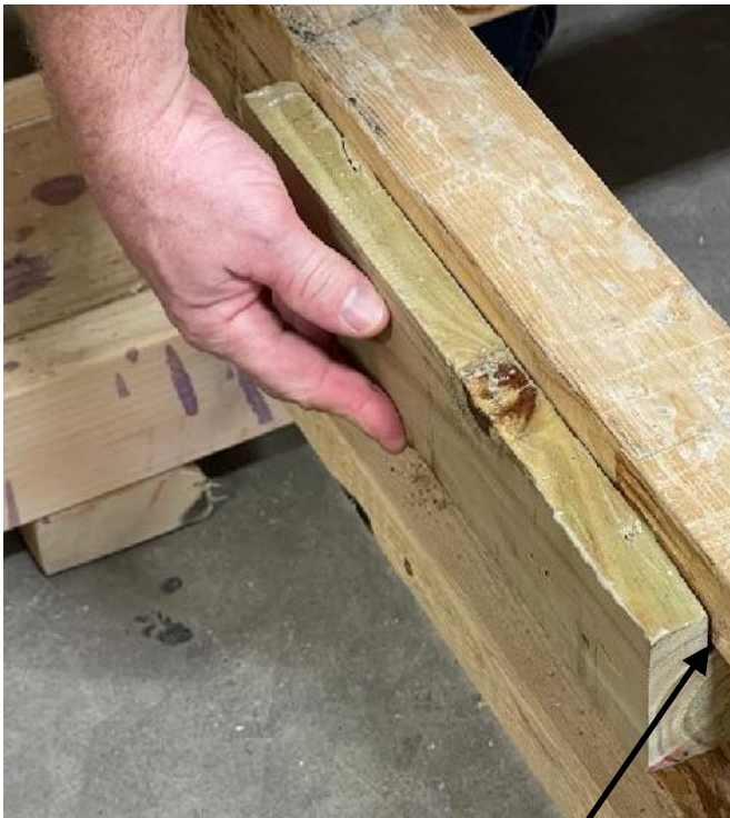
Notched drain support block cleat fits I-joist
