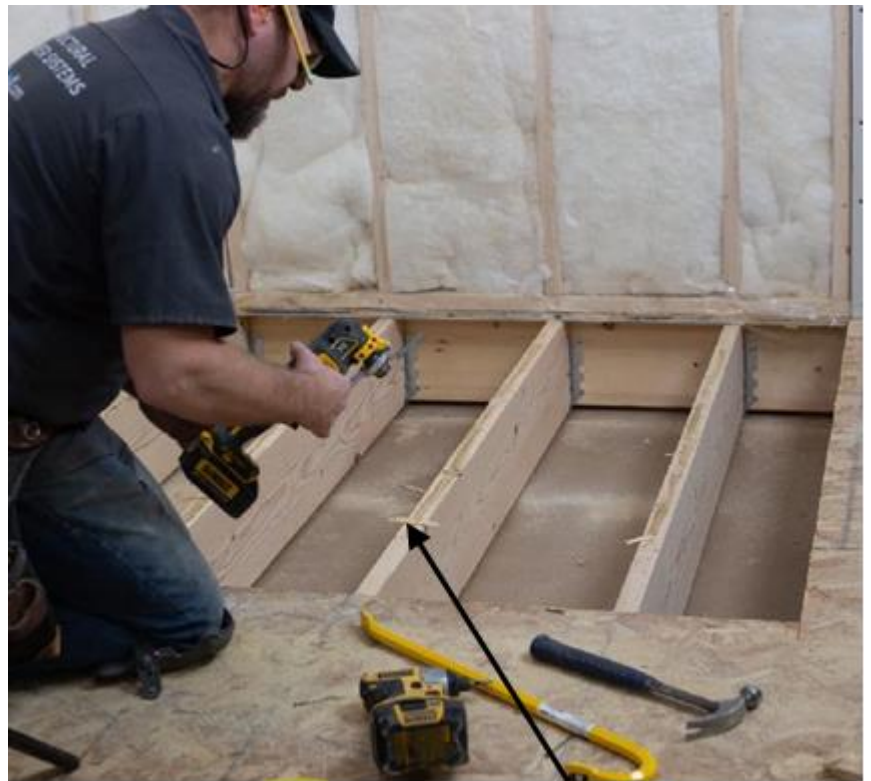
Clean top of joists with multi-tool
