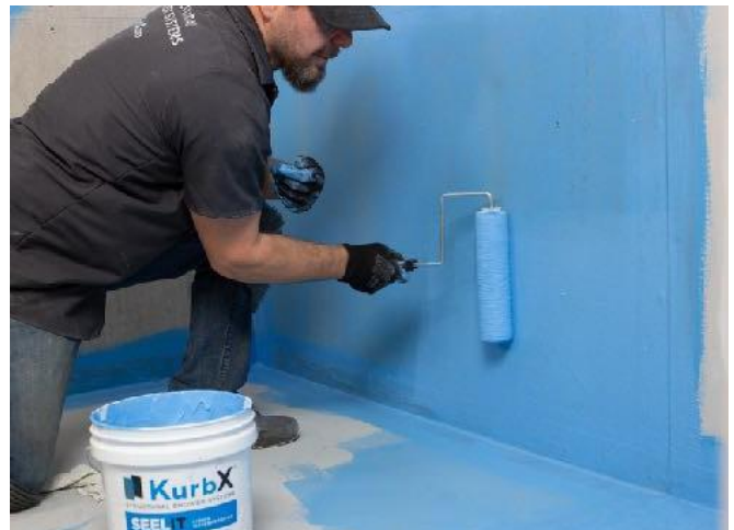
After 2 coats of waterproofing (not transparent) besides pan field
