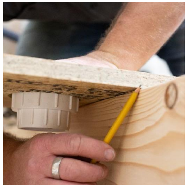
Trace bottom of drain support block along top of joists
