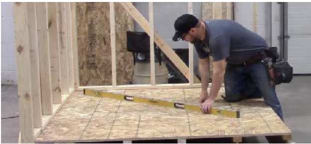
Check subfloor for level & flatness
