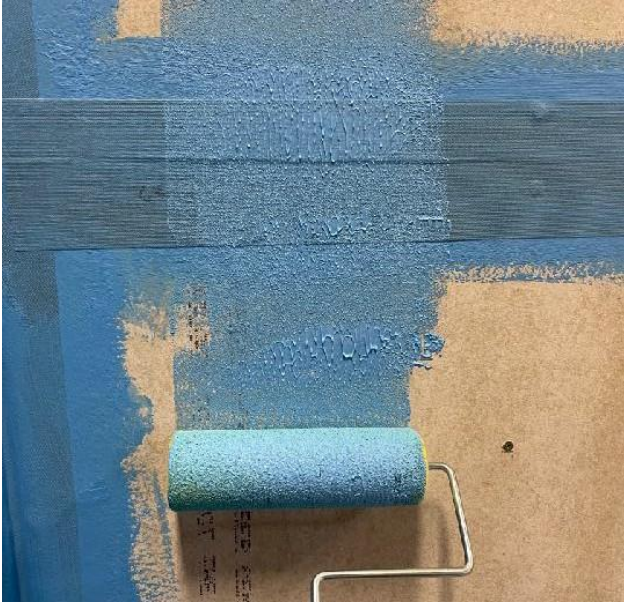
Apply the first coat in either a vertical or horizontal direction
