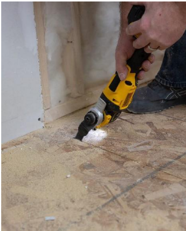
Finish cuts with multi-tool
