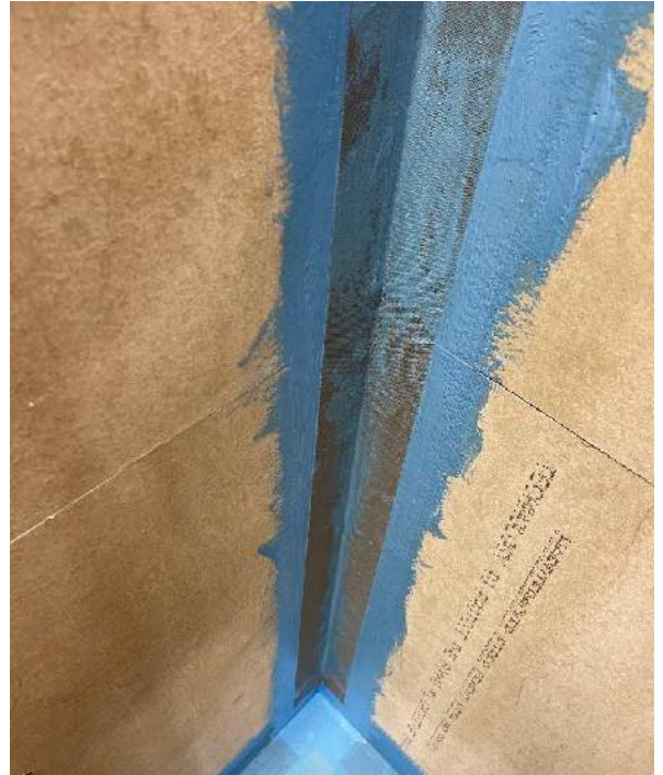
Vertical inside corner embedded
