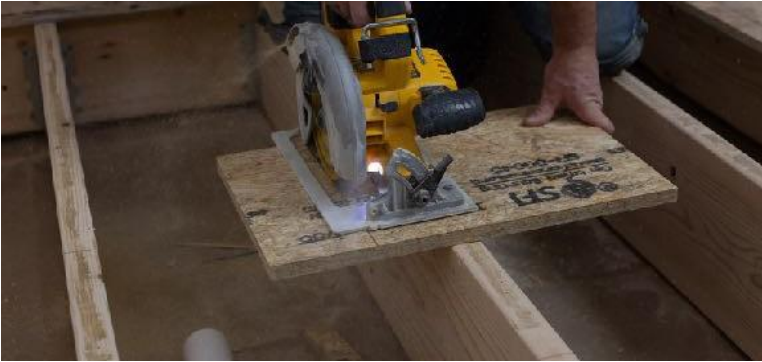
Cut drain support to length using the traced lines
